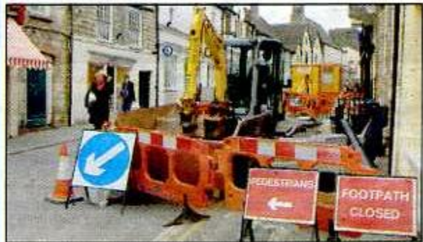
The roadworks in Long Street last week GSR240H10
